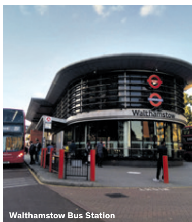
Walthamstow Bus Station
