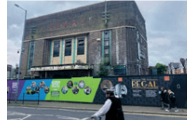
The Regal Cinema in Hale End Road pictured before works began
